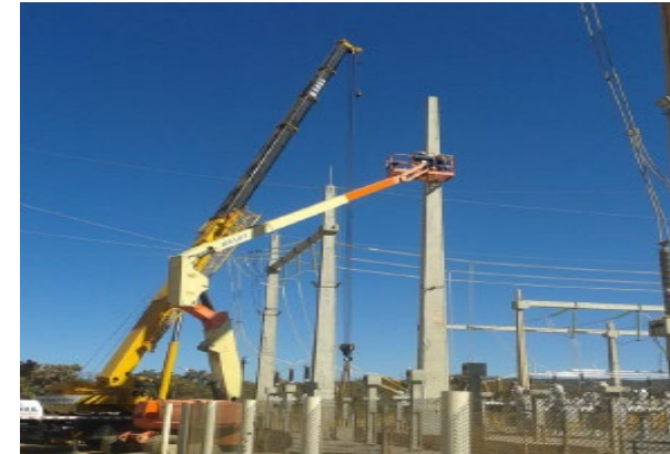
JMM. Substation Igarorã III 230Kv Installation of access gantry
