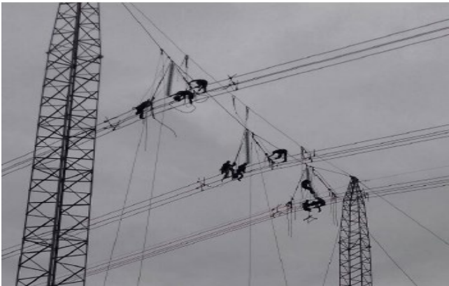
Odoya 500Kv – Sapeaçu – Morro do Chapéu II Conductor cable stapling
