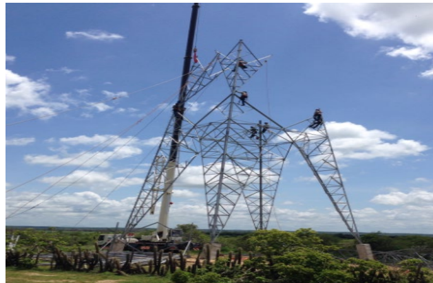
Esperanza. 500Kv – Quixadá II – Açú III Assembly of self supporting tower
